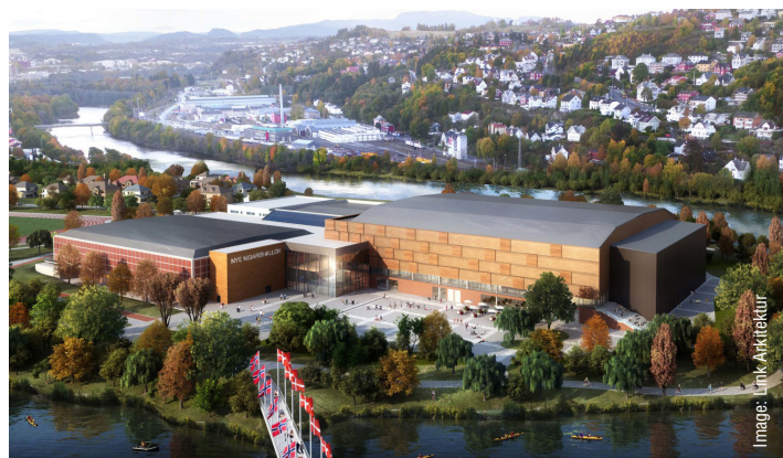
Trondheim is getting a new multi-functional sports centre called Nye Nidarøhallen. Bravida subsidiary Oras is planning and installing all heating and plumbing, HVAC and building automation solutions for the project. The new facility will accommodate everything from local amateur sport and various trade fairs to concerts with 12,000 visitors. The venue is estimated to be completed by autumn 2019.
