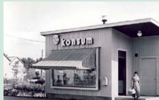
The first Konsum store is created and we contribute to the construction process.
