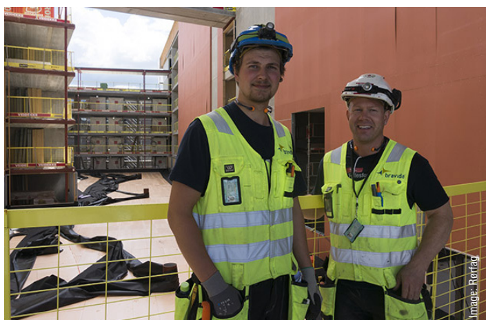
Vitaminveien 11 is currently under construction in Storo, Oslo. The area will house a hotel, apartments, offices, cinema theatres, parking spaces and a preschool. Together, the new buildings will comprise an area of 62,000 square metres. Orders for all the heating & plumbing installations are worth NOK 70 million and Bravida is working with Rørtema AS to carry out the installations. The project is expected to be completed in 2019.
